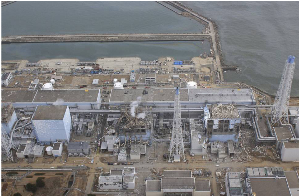
Figure 3. Fukushima Dai-ichi following destruction of reactor building superstructures due to hydrogen explosions (source unknown)
